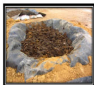
Figure 5 Soil treatment with Enretech-1 and water
